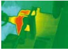
Motor: Bearing Problem
